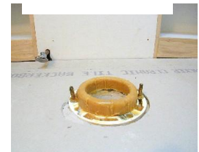
Figure 8: New wax ring.
