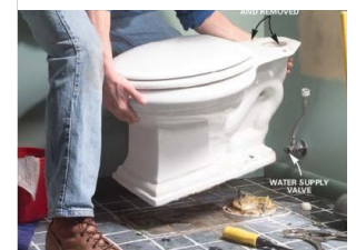
Figure 4: :Lifting the toilet.
