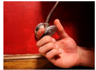
Figure 1: Water Stop (water valve or angle)
