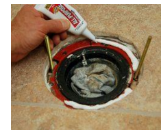
Figure 7: Caulking the new flange.
