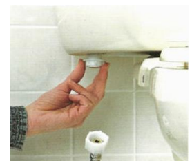
Figure 2: Removing the jam nut
