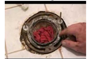
Figure 6: Checking the old flange.
